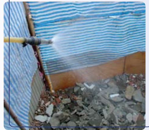
Water spraying at refuse storage to reduce dust 廢物收集站設有灑水裝置以減低塵埃
