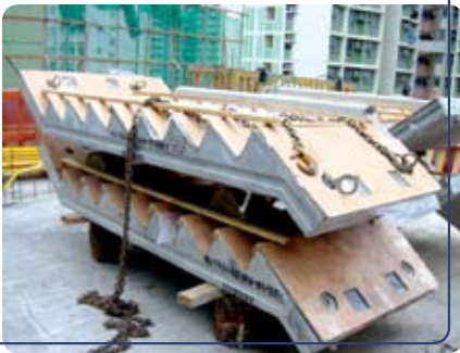
Prefabricated components for construction 預先製成的建築組件
