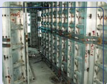
Aluminium formwork for construction 建築用的鋁質模板
